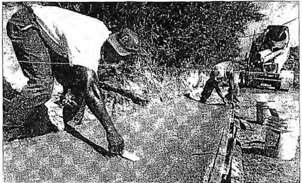
Island Roads workers Raphael Victor and Odirgo Jose prepare a concrete drainage gutter Friday afternoon along Mandahl Road on St. Thomas
